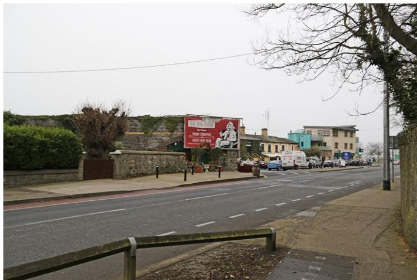
Plate 15: Northern side of tram viaduct with Howth Station at rear
