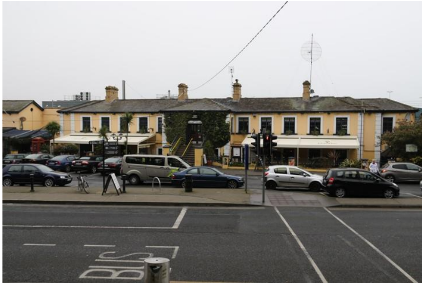
Plate 9: Howth railway station
