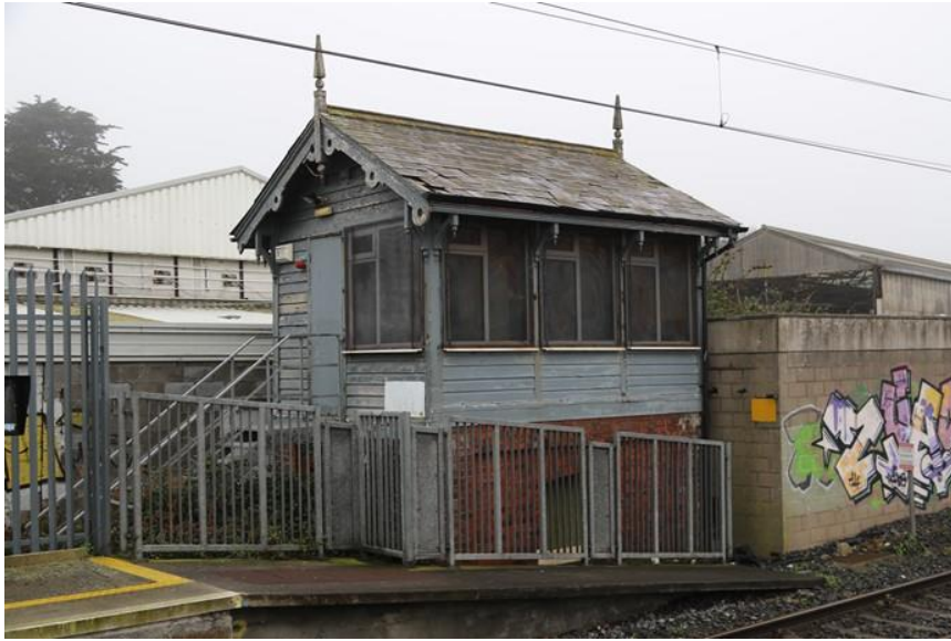
Plate 11: Signal box at Howth Railway Station
