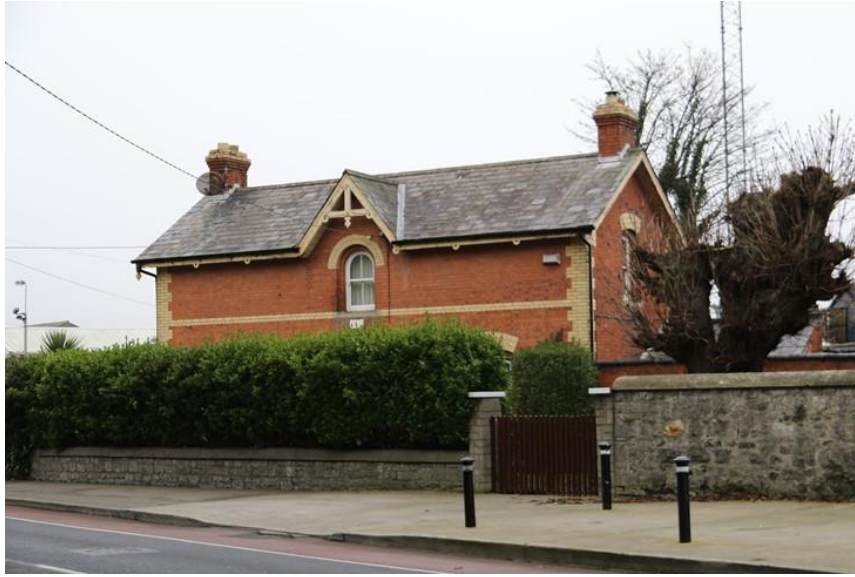
Plate 7: Station master's house
